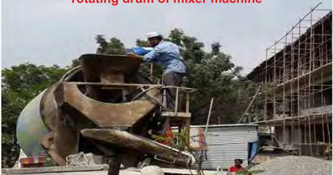
Figure 4: View of addition of Polymer in the rotating drum of mixer machine
